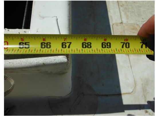
Remove skylight, or measure curb only, not skylight frame
