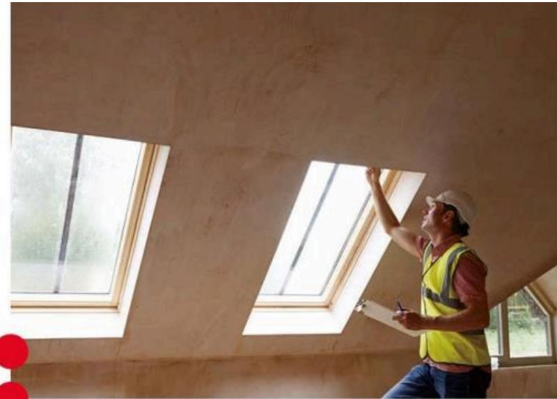
Testing should be performed as soon as possible after the skylight is installed, and prior to the installation of drywall or other interior finish materials.
