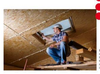
Be aware that after the rough opening has been prepared, per the manufacturer's dimensions, temporary support of the rafter may be necessary if a rafter is cut.
