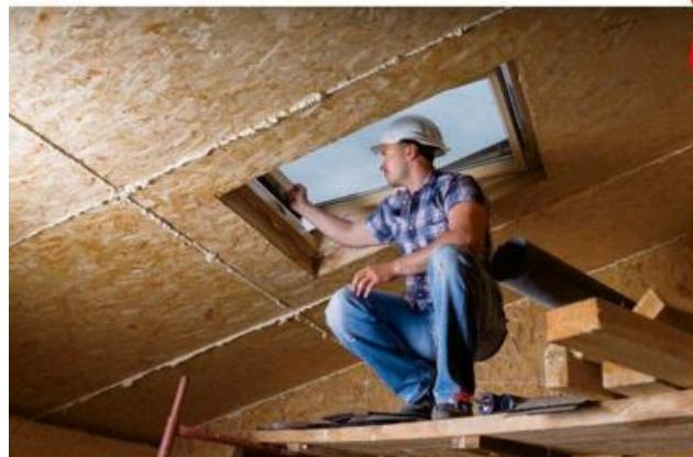
Be aware that after the rough opening has been prepared, per the manufacturer's dimensions, temporary support of the rafter may be necessary if a rafter is cut.
