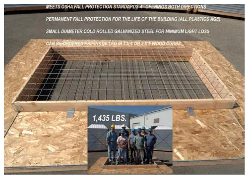
during the lifetime of the opening. Utilizing an exterior mounted device for fall protection becomes an issue at the time of roof replacement or reroof when the dome and exterior device need to be removed in order to perform flashing details. Once removed, the opening is no longer in compliance with the regulation and as such, the roofing contractor is required to protect the opening
