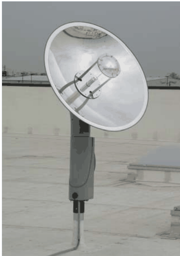
Hybrid Solar Lighting tracking sunlight collector with parabolic primary mirror
