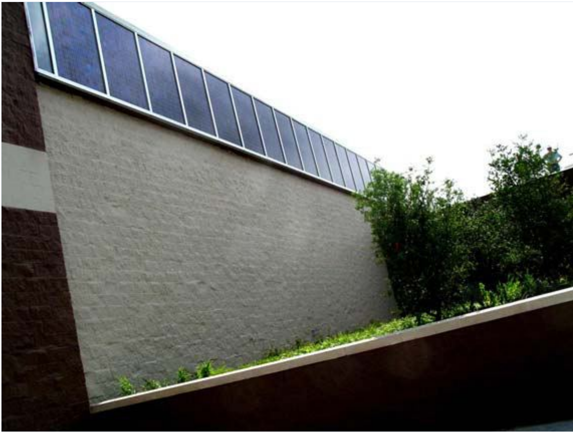
PV Array 5 blue stripe polycrystalline modules extending beyond the clerestory glazing
