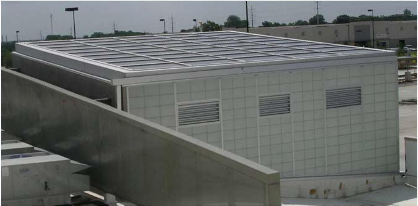
Roof and top of one of the entrance vestibules (PV Arrays 1 and 2), showing translucent siding and vent louvers
